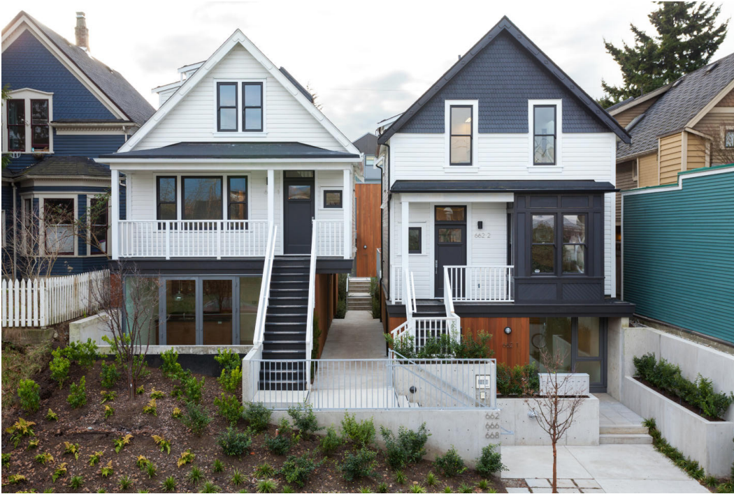
Figure 13 Union Street Eco Heritage, high density within a conventional and contextual mass and ornamentation
