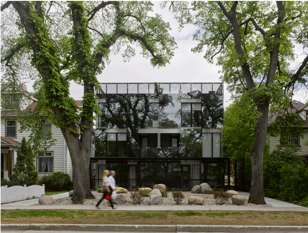
Figure 15 548 Stradbrook, illustrating the continuity of the built form at the street despite the differential typology and aesthetic treatment.
